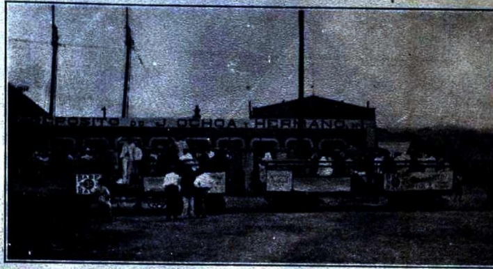
PLATFORM TRAILERS FOR SUNDAY TRAFFIC
