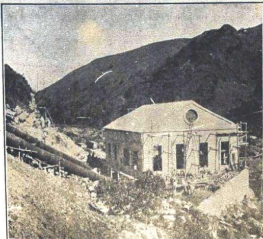
COMERIO FALLS POWER PLANT, NEARING COMPLETION
